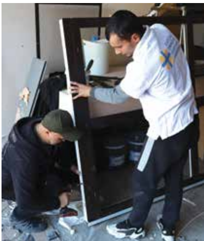
A Caritas Ukraine team repairing windows.
