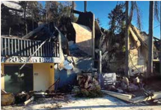
Anna Maistrenko's apartment building in Pacific Palisades after the fire.
